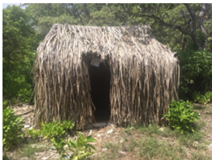
Toilet Facilities at Ueen Abaiang JSS
