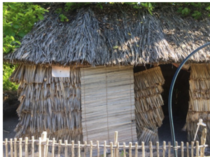
Toilet Facilities at Tanimaiaki Primary School, Abaiang
