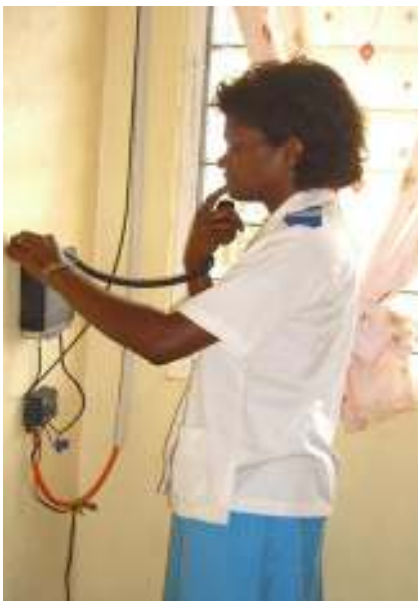
Dogotuki Nursing Station (Cakaudrove, Vanua Levu) was upgraded in 2006 but while there are light bulbs there is no electricity. At night, the sole nurse must attend to emergencies or deliveries using a kerosene light. Her only way to contact medical help is by a fitful radio telephone and her main means of transport is by foot.
